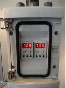
Single Channel pH Controller 3TX-2M-pH-A-REL
